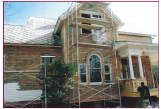
Terry Hayes' Restoration, exterior paint removal (using the #1 Paint Stripping System by Speed Heater)
