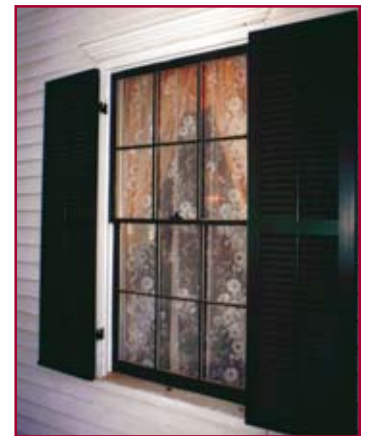
Window restoration at Knott House
