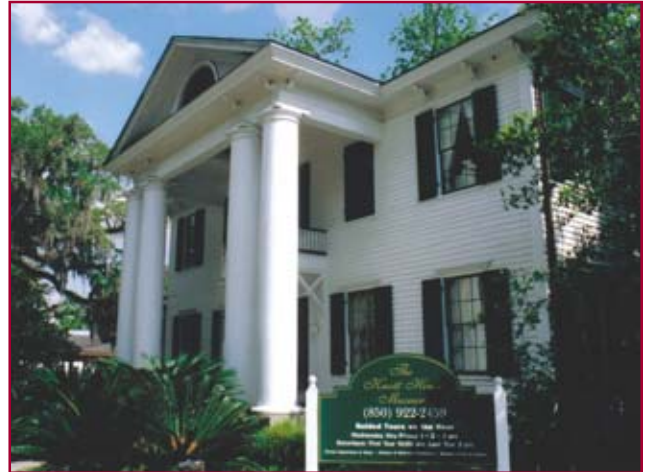
Knott House Museum 1843, Tallahassee FL, Window and shutter restoration
