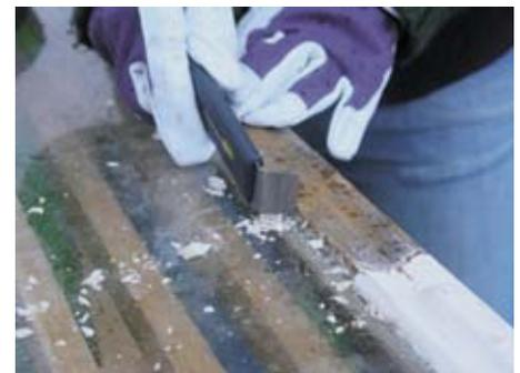
Scrape of residual putty from glass with the putty scraper. Speedheater Systems Putty scraper is specially sharpened not to scratch the glass.
