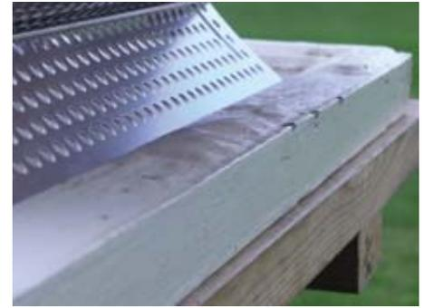
Place the Speedheater 1100-15 in an angle with the help of the angle support. Begin heating paint and putty for about 1-2 minutes. Putty takes a little longer to soften than paint and even if the paint surface is ready and it has bubbled up, it is good to wait close to 2 minutes for the putty to soften.
