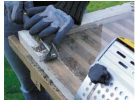
Move Speedheater 1100-15 to the next area and begin heating. Use the Boomerang Scraper with both hands and remove all layers of paint from window frame. The Boomerang Scraper is also great to use when removing paint from fine carpentry and detail.
