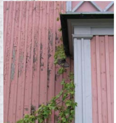
Their first thought was that the paint used on the house was of poor quality but they were mistaken. Sample tests of the surface showed that there was an active ingredient common in chemical strippers.
